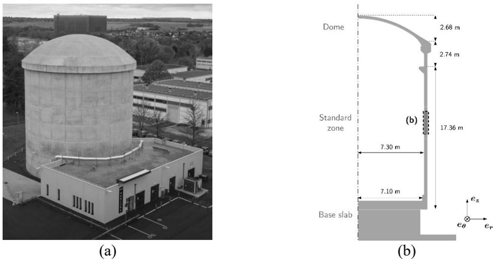
372 *Figure 10: Experimental 1:3 scaled double-walled nuclear containment building (NCB) – VeRCoRS mock-up:*
